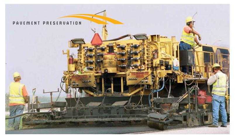
"We overlapped two to three inches of the previous repaved lane to make sure we had a clean bond between the two travel lanes," says Don Allensworth, Cutler paving superintendent who is in charge of the I-29 repaving work.
