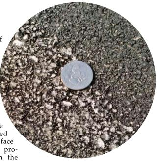
Above is an example of the "seamless" joint between lanes after compaction.
