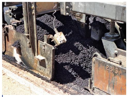
The paver can be augmented to any width needed via a series of pre-made, 1-ft extensions for the heating hood, scarifying teeth and the recycling auger. This adaptability allowed Cutler to set a new Arizona record with one pass of 18 ft.
