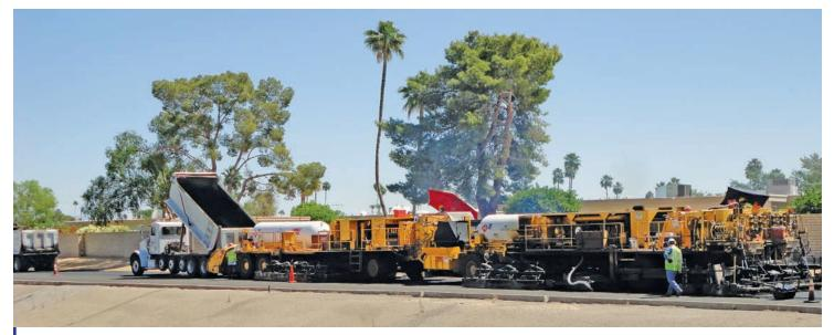
Cutler brought in its own paver. Going one lane at a time, the machine heated, scarified and recycled the top layer, refreshing it with new asphalt emulsion. While the recycled layer is still hot (at least 200°F), an additional inch of fresh material is placed on top.
