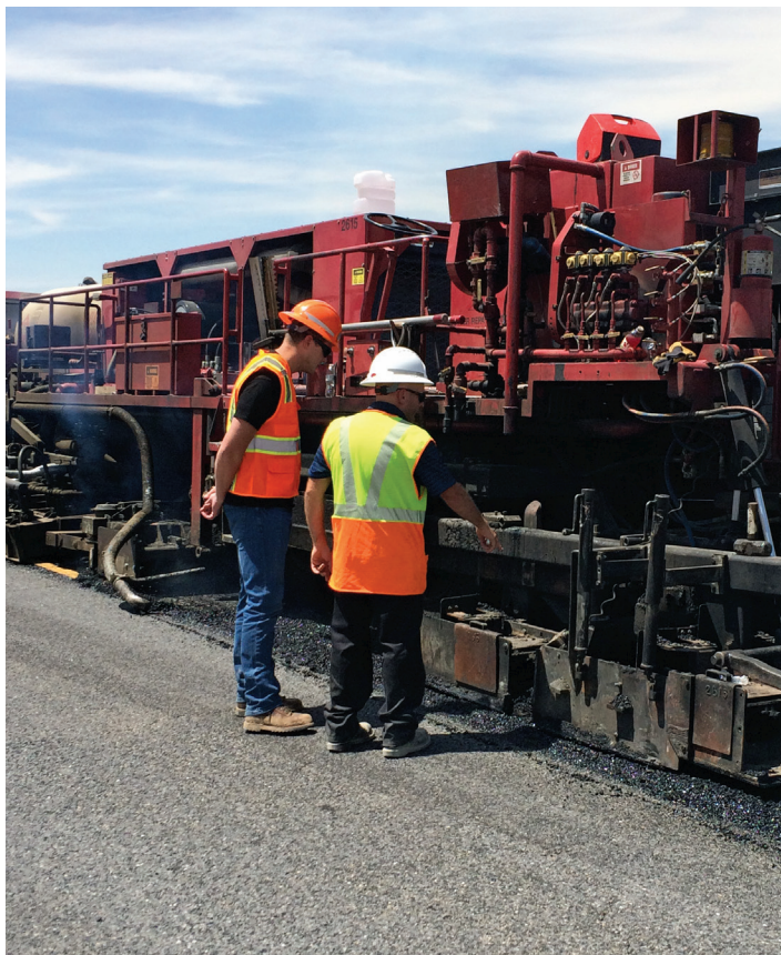
Crews check the progress on the paving train, which was led by a pair of propane heaters that allowed the R-2100 preheater conveyor vehicle to get the material immediately ready for reclamation, mixing and reapplication.
