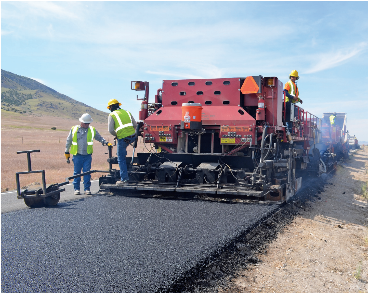
The new wearing course is laid immediately after the recycled layer for a monolithic bond.
