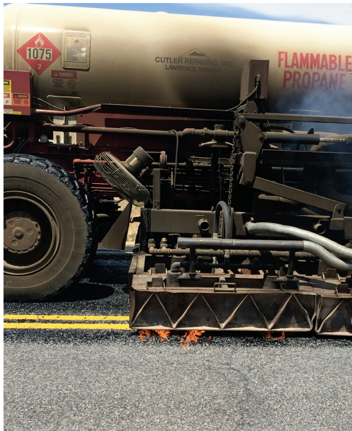
Crews check the progress on the paving train, which was led by a pair of propane heaters that allowed the R-2100 preheater conveyor vehicle to get the material immediately ready for reclamation, mixing and reapplication.
