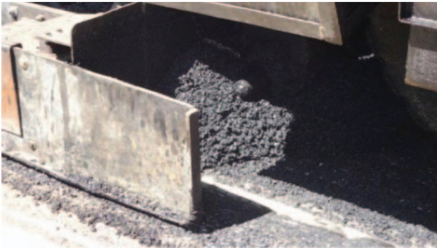
This photo shows the recycled material being placed by the screed on the repaver. This material has essentially the characteristics of new AR mix due to the restoration of the mix during the recycling process.
