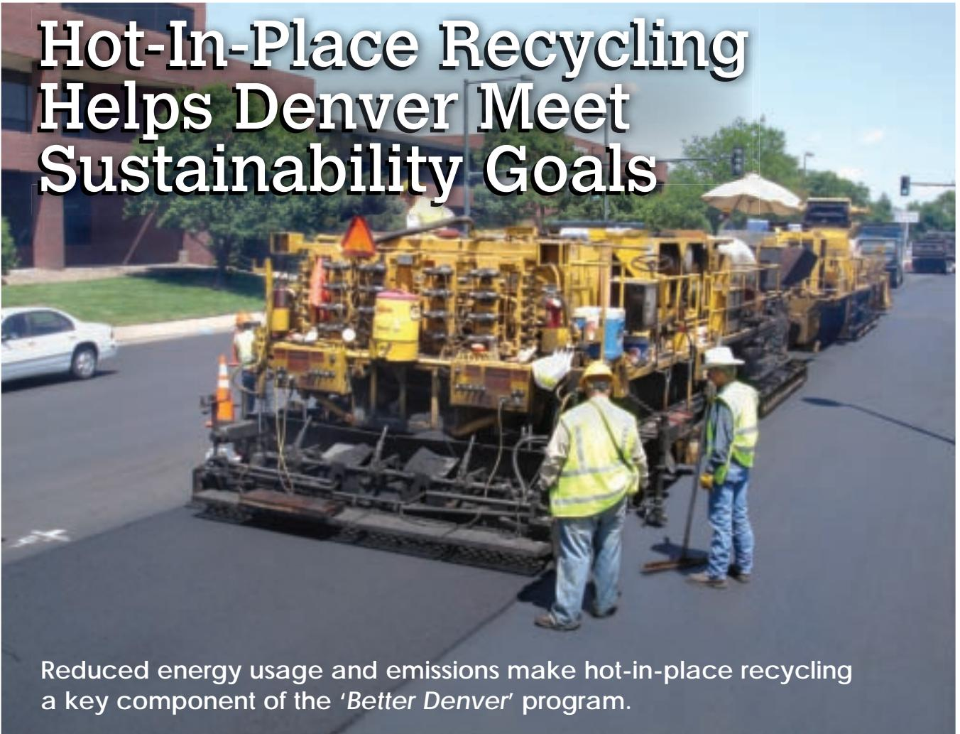
Reduced energy usage and emissions make hot-in-place recycling a key component of the 'Better Denver' program.
