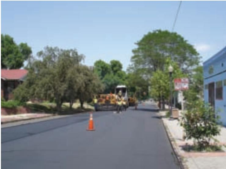
Denver enhances the sustainability of its repaving program by using up to 40 percent reclaimed asphalt pavement in the hot-mix wearing course.
