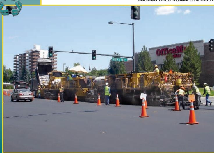
Cutler's single pass recycling process completes the recycling and resurfacing simultaneously, thereby minimizing delays to the traveling public.
