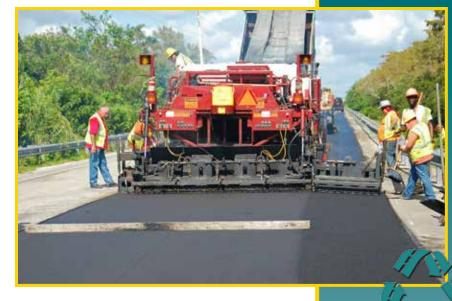
To place a final friction or driving course, other hot in-place processes use a separate paver following the heater/scarification process. But Cutler uses a screed at the rear of the repaver and thus is able to eliminate an entire machine.
