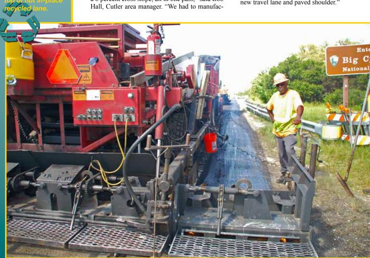
Repaving Inc. built bolt-on screed extension to permit virgin HMA paving of 4-ft. shoulder with 6 percent cross slope in conjunction with virgin paving of 12-ft. driving lane with 2 percent cross slope immediately on top of hot in-place recycled lane.
