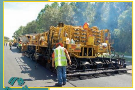
Hot in-place recycling with the Cutler Repaving process helps keep county PCI high.
