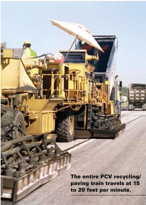
**The entire PCV recycling/paving train travels at 15 to 20 feet per minute.**
