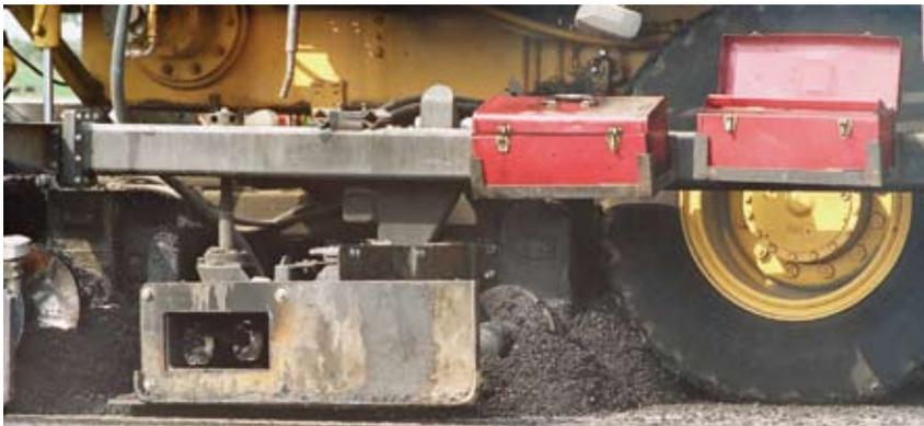
**The top photo shows the one-pass asphalt recycling method in action. The middle photo shows the recycling agent being applied and mixed, while the bottom photo shows the recycling screed laying the recycled mix.**
