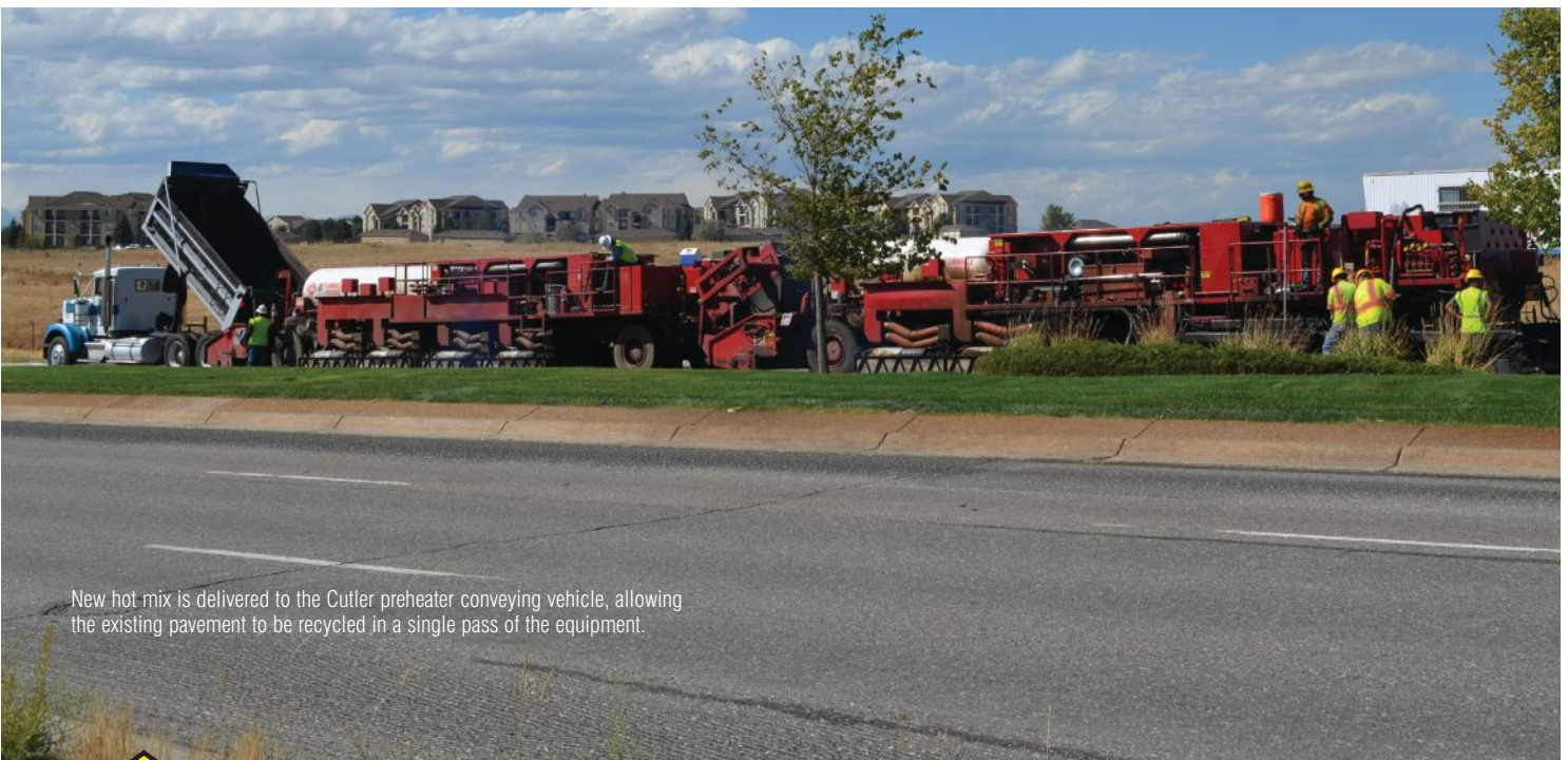
The existing pavement is recycled and resurfaced in a single pass of the Cutler Repaving equipment, thereby minimizing traffic delays.
