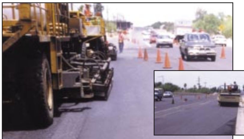
Two views of the HIPR process of Flowing Wells Road, Pima County, Arizona
