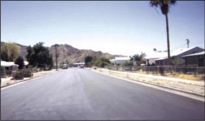
Two-lane suburban road in Ajo, Arizona resurfaced by Cutler Repaving
