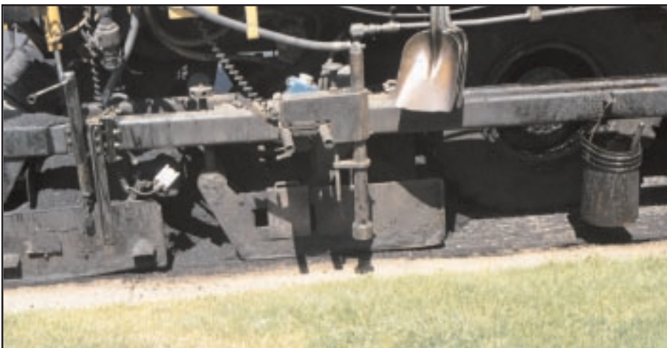
Reclaimed asphalt is reapplied and distributed with a screed as a 1 inch leveling course
