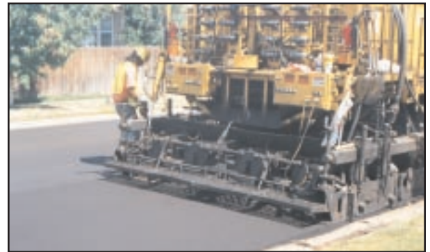
Vibratory screed applying new HMA overlay
