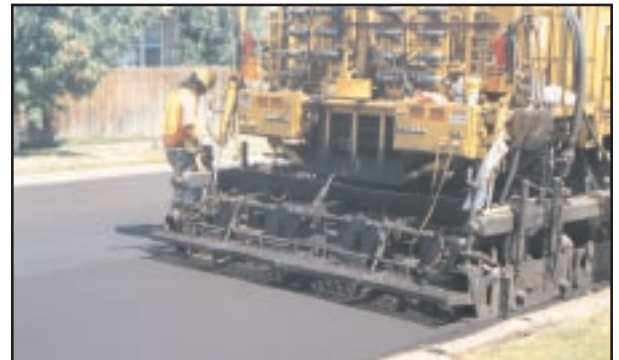
Vibratory screed applying new HMA overlay
