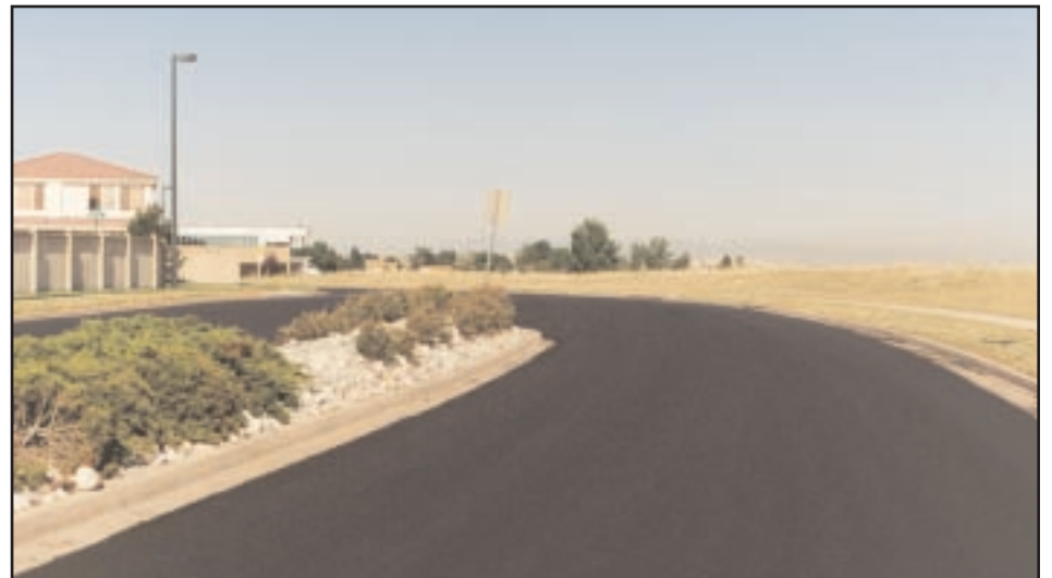
Cutler's Repaver works well on streets with tight curves
