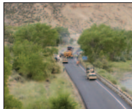
Elimination of longitudinal joint produces smooth process.
