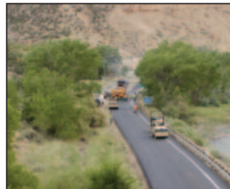
Elimination of longitudinal joint produces smooth process.
