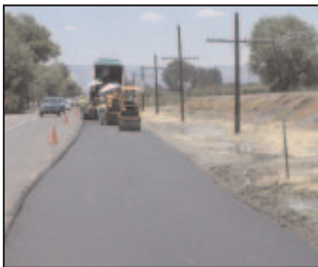
One-pass repaving keeps work zones compact, traffic flow smooth.
