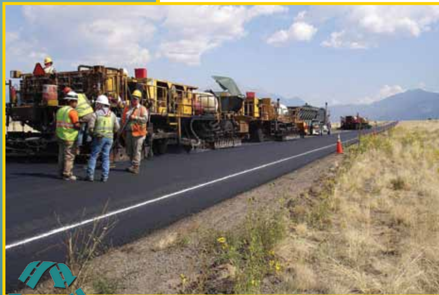
Hot in-place recycling (HIR) train on Colorado S.H. 150 included, from left, repaver, preheater, virgin HMA haul unit for surface course, and auxiliary preheater.
