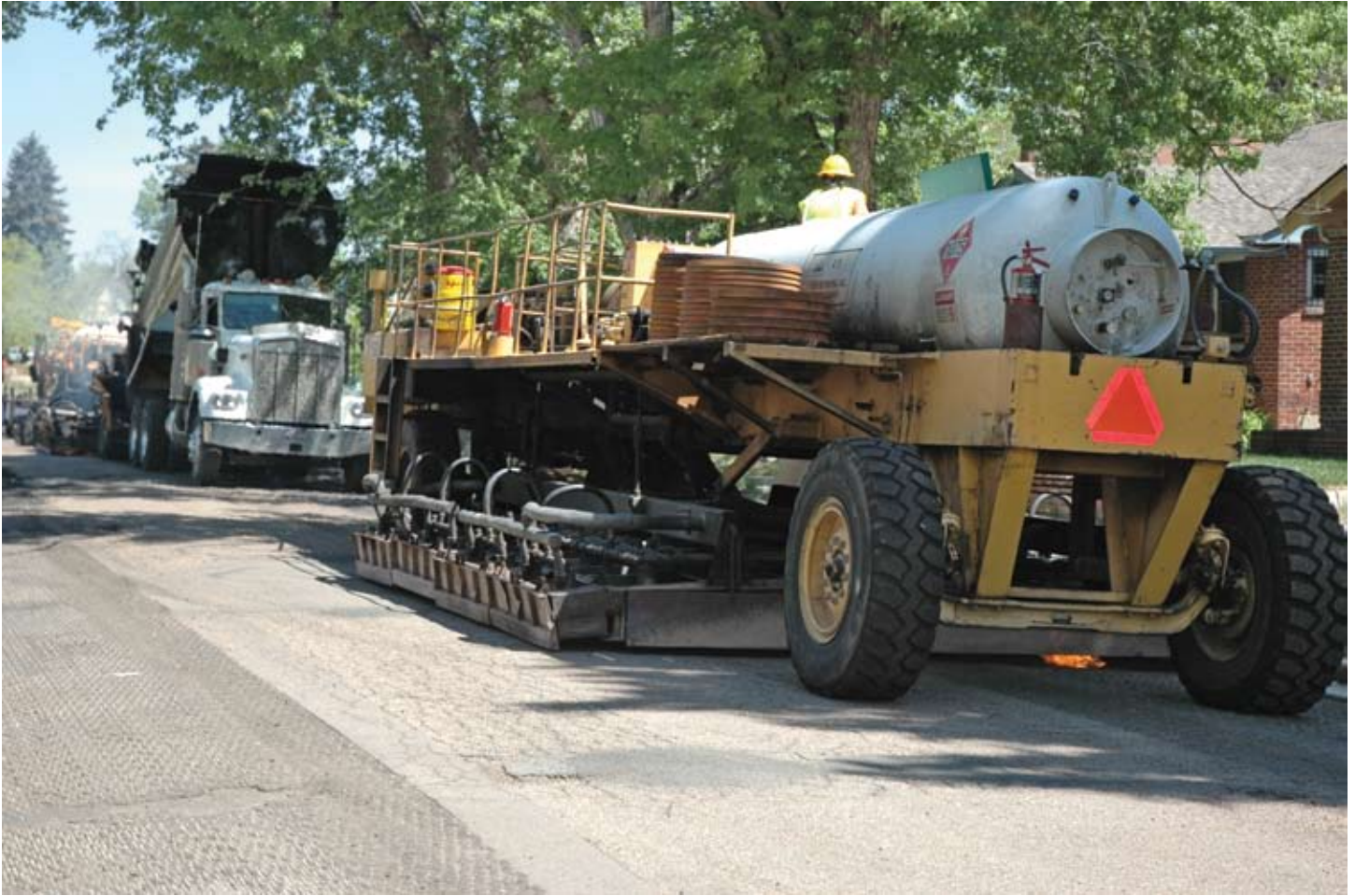
Cutler's exclusive repaving process heats the existing pavement to 300 degrees F. Once softened, the pavement is scarified to a depth of 1 inch and then a rejuvenating agent is added to restore the viscosity of the aged asphalt.
