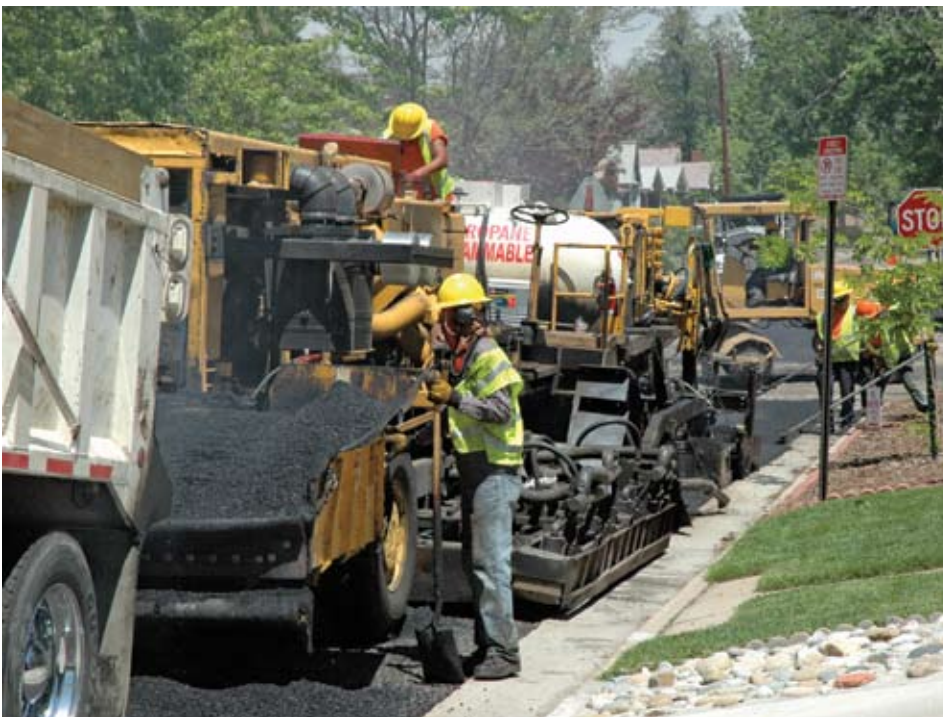
Cutler's exclusive repaving process heats the existing pavement to 300 degrees F. Once softened, the pavement is scarified to a depth of 1 inch and then a rejuvenating agent is added to restore the viscosity of the aged asphalt.
