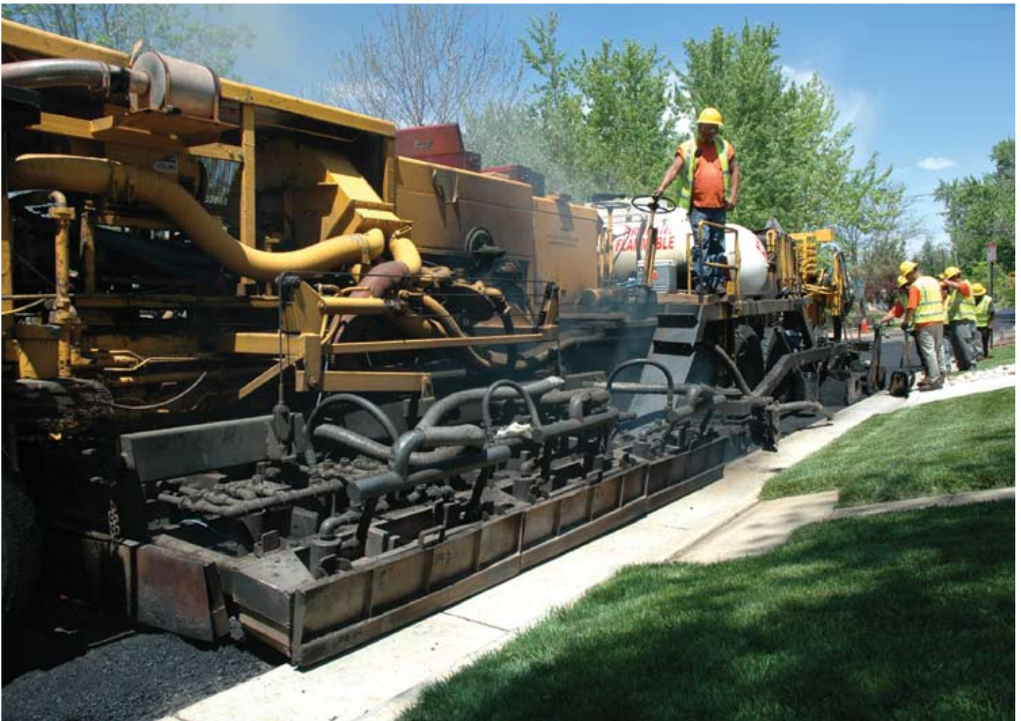
Heating, scarifying, applying rejuvenating agent and applying new overlay is done in a one-pass process with the proprietary equipment Cutler uses. The process delivers a high-quality road with fewer disruptions at a lower cost than conventional mill and overlay roads.
