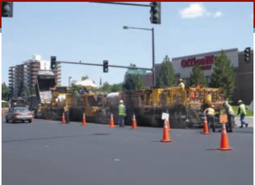
In Denver, hot-in-place process places HMA over freshly recycled base course.
