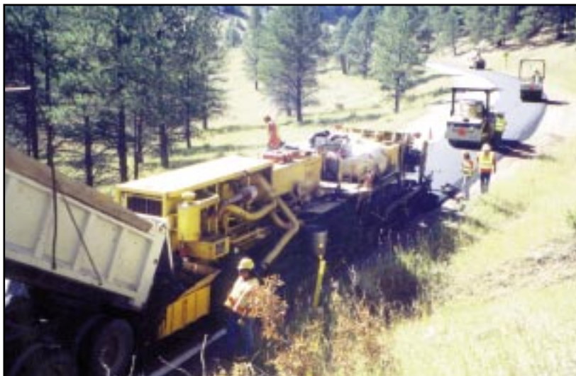
The machine travels quickly and lane closures are minimized. All reclaimed material is used on the spot without hauling and truck traffic is eliminated.
