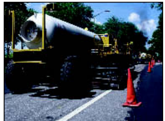
In Orlando, independent unit prebeats pavement ahead of main Repaver.
