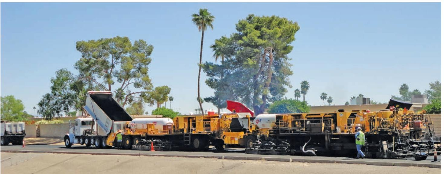
Cutler brought in its own paver. Going one lane at a time, the machine heated, scarified and recycled the top layer, refreshing it with new asphalt emulsion. While the recycled layer is still hot (at least 200°F), an additional inch of fresh material is placed on top.
