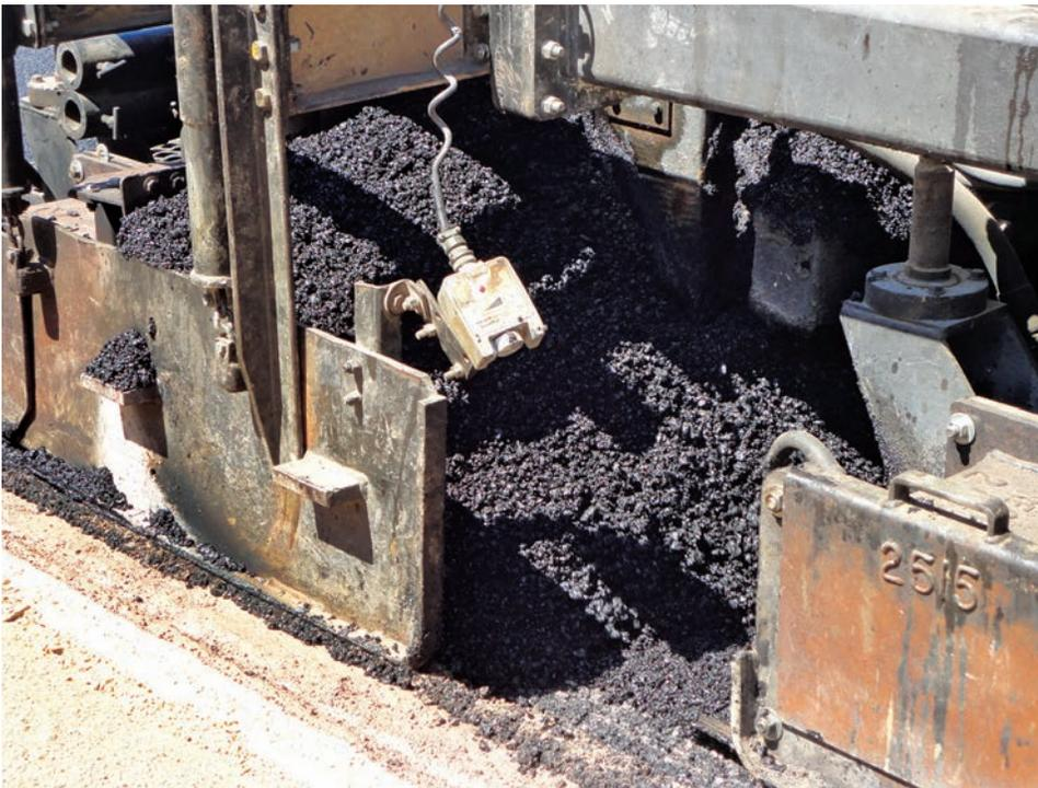
The paver can be augmented to any width needed via a series of pre-made, 1-ft extensions for the heating hood, scarifying teeth and the recycling auger. This adaptability allowed Cutler to set a new Arizona record with one pass of 18 ft.
